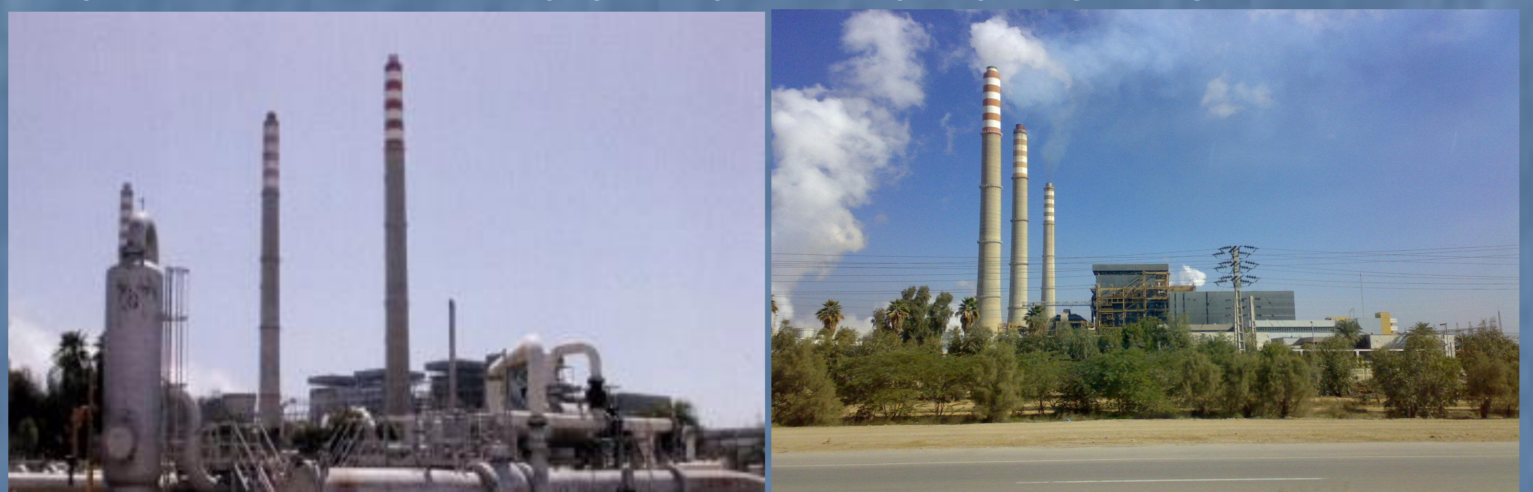
Figure 4. picture of Ramin power plant near Ahwaz
